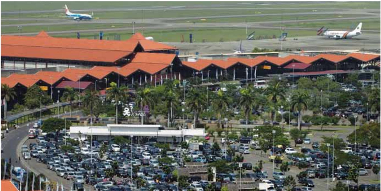
The terminals at Soekarno-Hatta Airport in Jakarta are already operating at levels in excess of their capacity.
